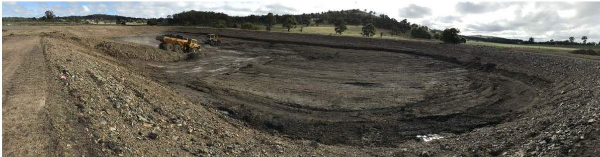
Figure 1 - Clay Lining of the Treated Effluent Storage Dam
