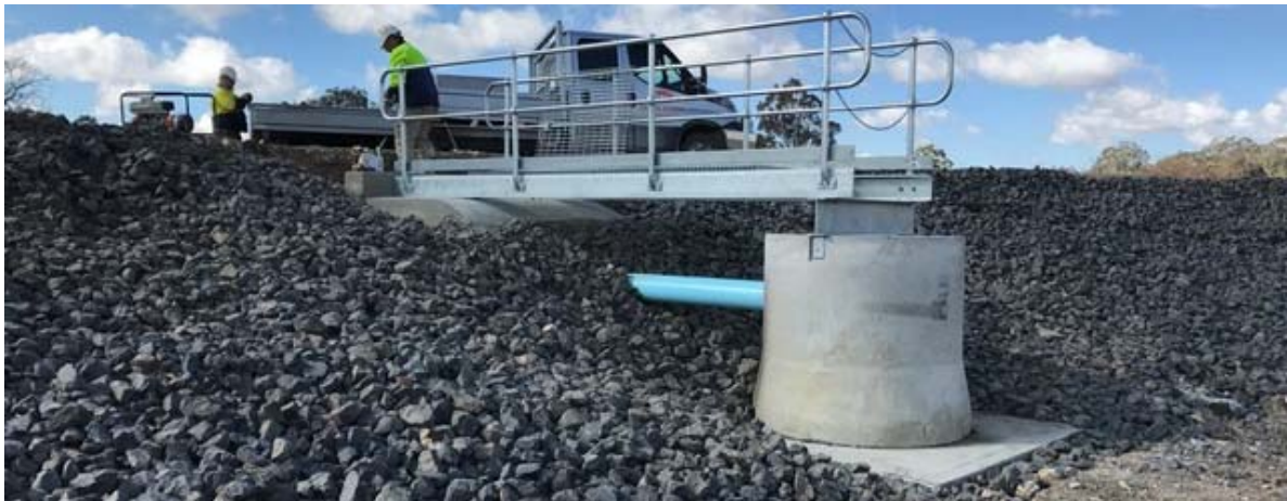
Figure 2 - Maturation Pond Access Walkway
