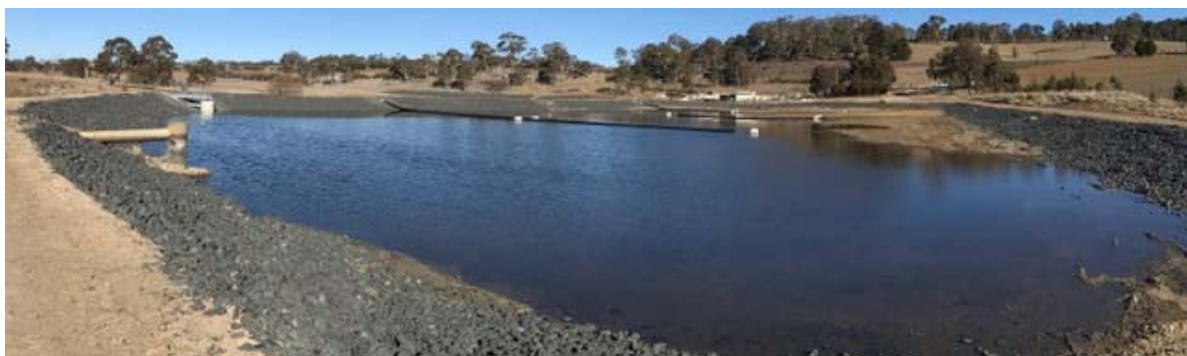
Figure 1 – Filling of Refurbished Maturation Pond
