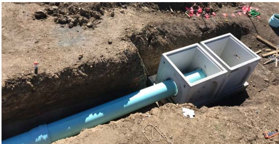
Figure 4 - Storage Pond Outlet Exterior
