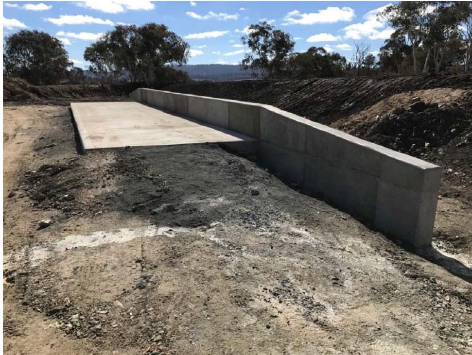
Figure 3 - Skip Bin Slab & Retaining Wall
