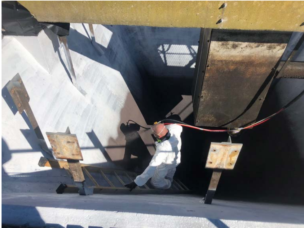
Figure 1 – STP Sedimentation Tank undergoing repairs
