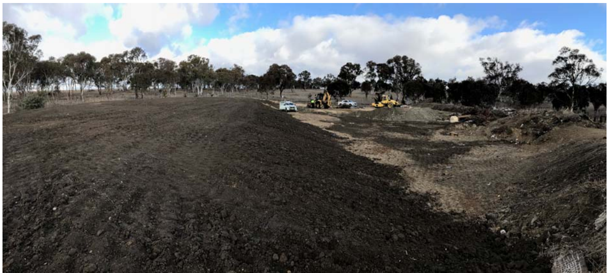
Figure 1 – Waste stockpile now capped
