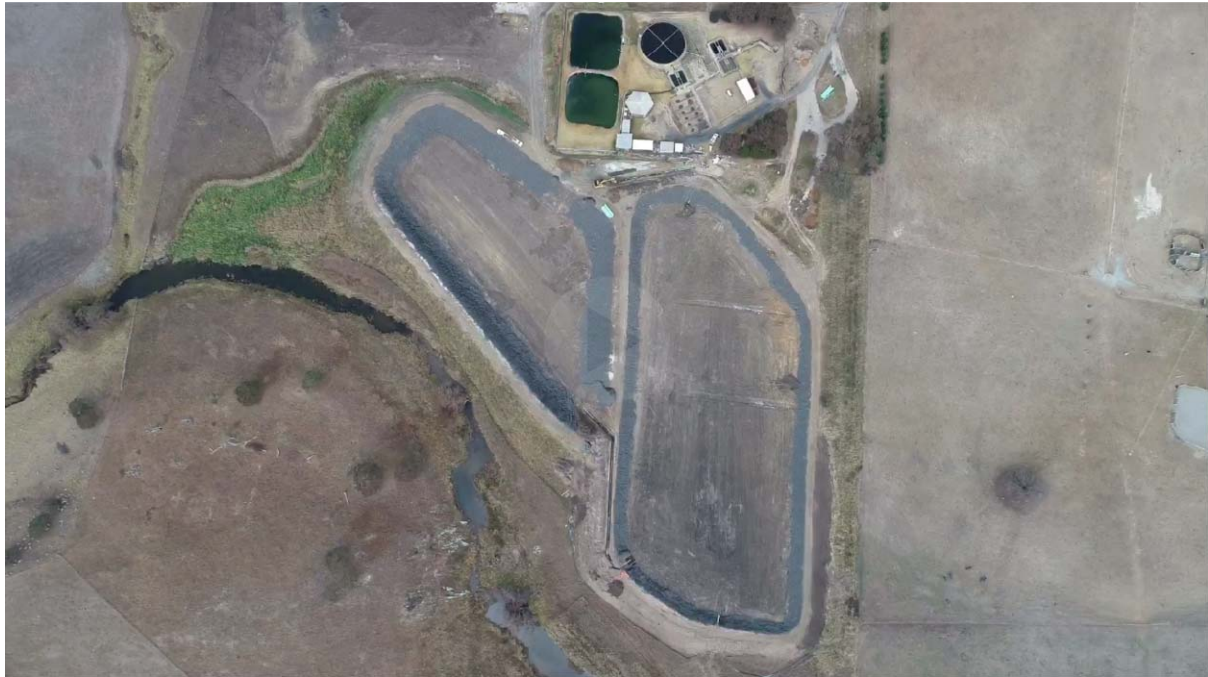
Figure 3 – Storage Dam and Maturation Pond
