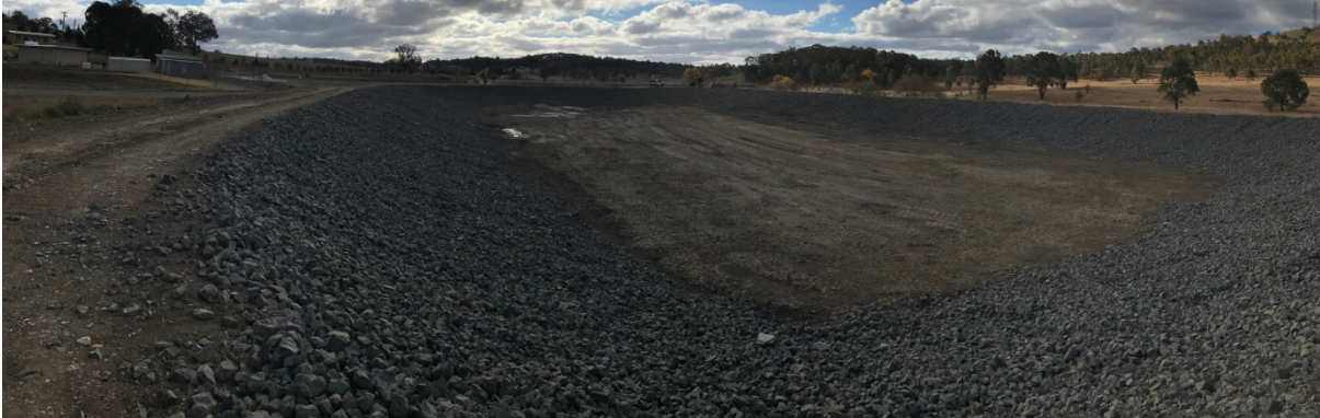
Figure 1 - Effluent Storage Dam
