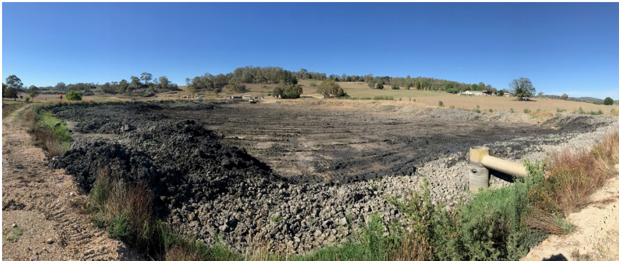
Figure 2 - Maturation Pond Sediment Stockpiling
