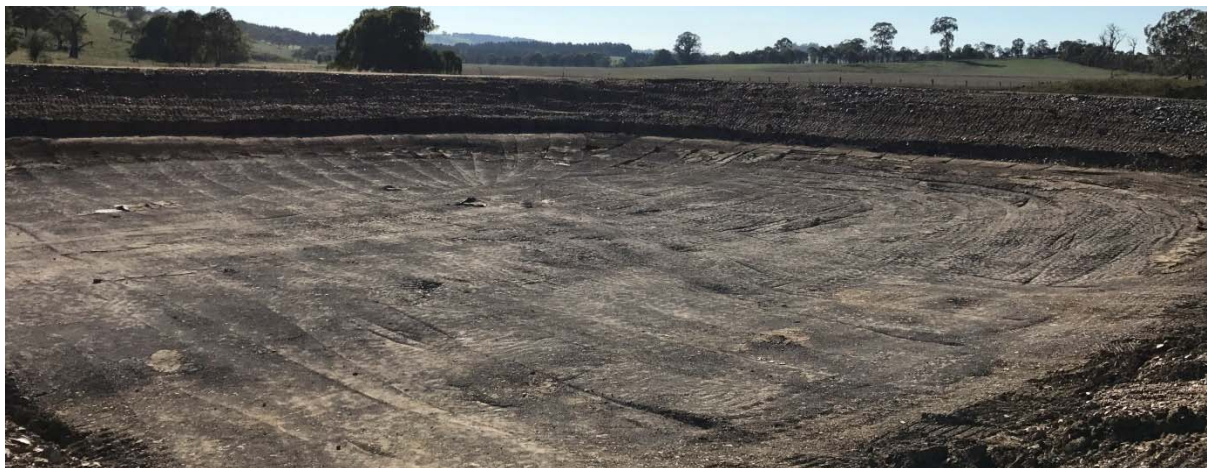
Figure 1 - Clay Lining of the Treated Effluent Storage Dam
