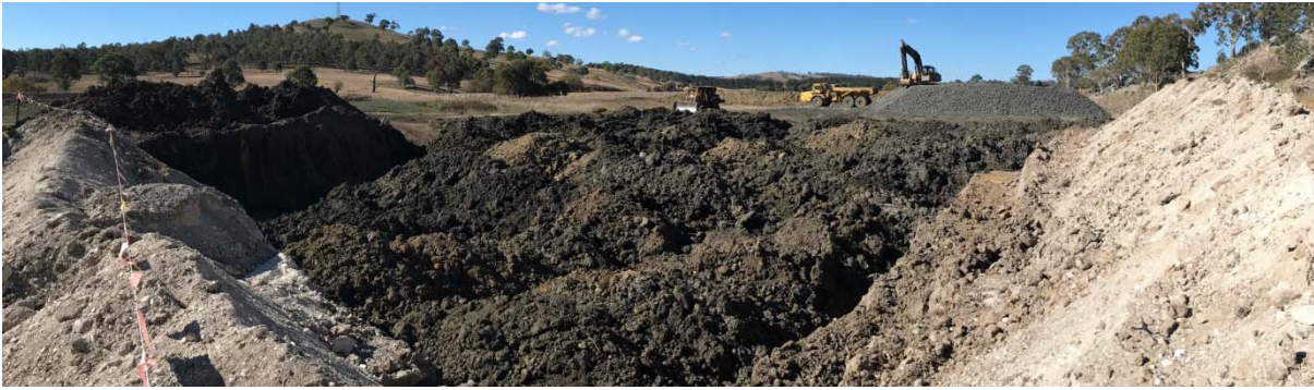
Figure 2 – Clay Pit/ Biosolid Storage Area
