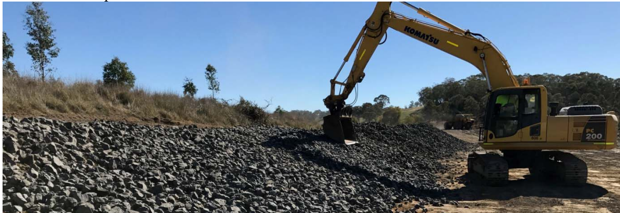
Figure 3 - Gabion Lining of the Maturation Pond
