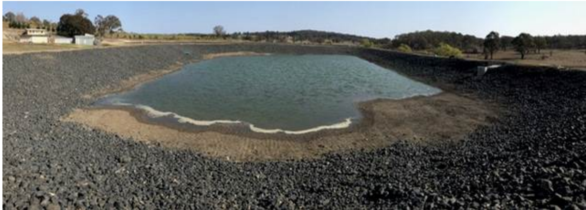
Figure 9.8.4 - Storage Pond Filling in Progress
