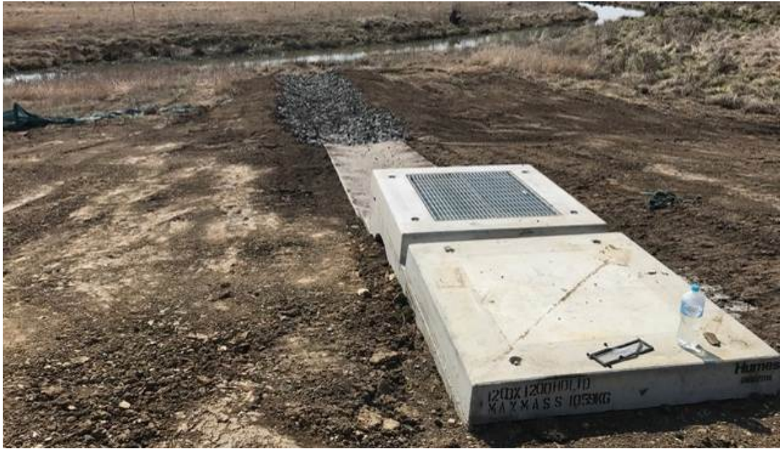
Figure 9.8.2 - Storage Pond Outlet Exterior – discharge point to the Apsley River
