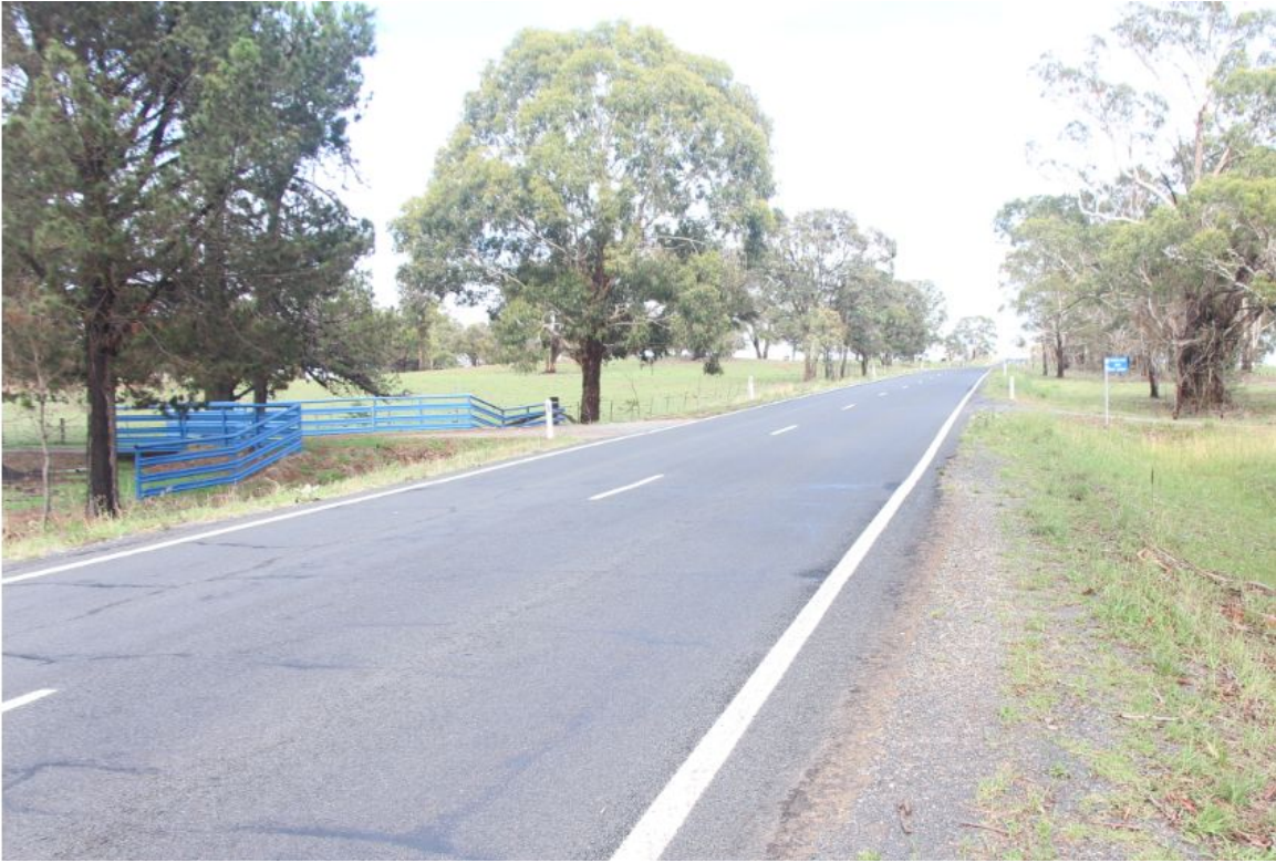
Plate 1 – Existing “Brooklyn” access road, left side of Oxley Highway 19-1-2020 (looking west).
