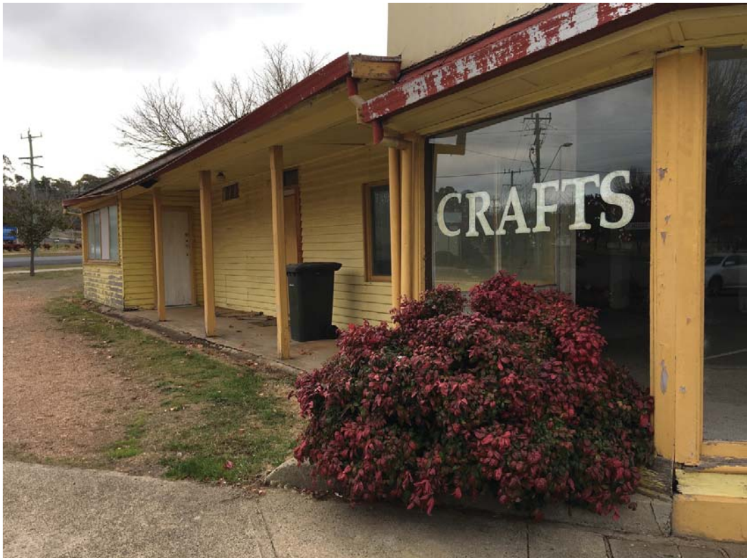
Shopfront window and verandah (Image: Studio Two Architecture 26/06/2019)
