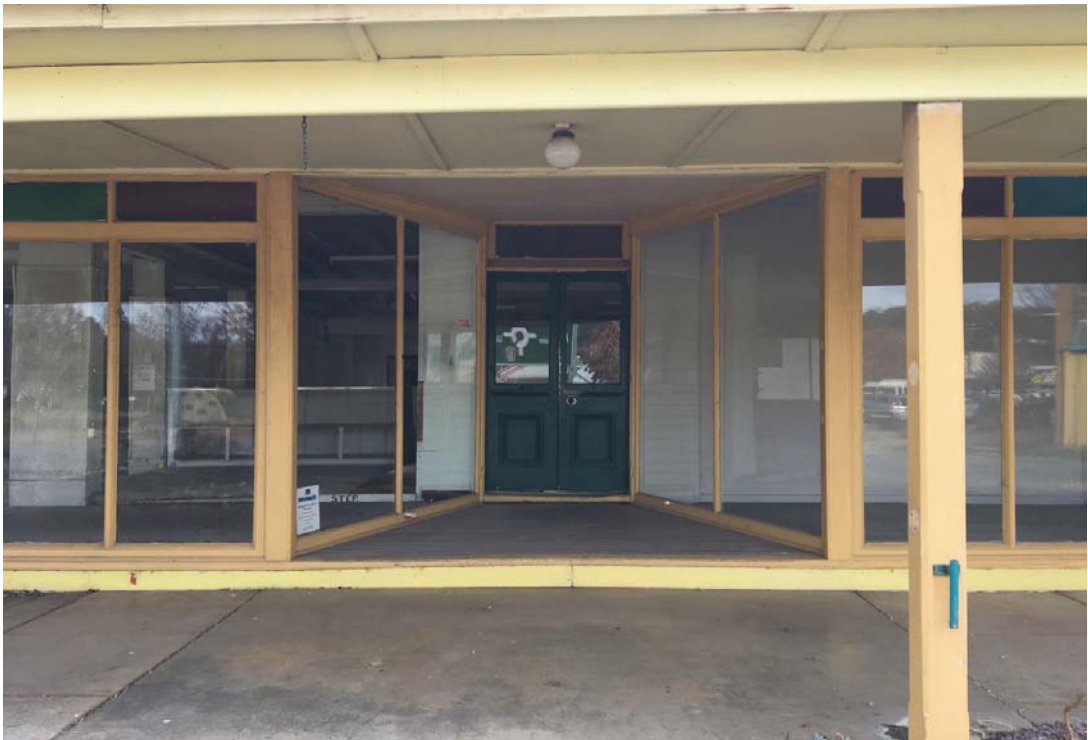
Shopfront window and entrance (Image: Studio Two Architecture 26/06/2019)
