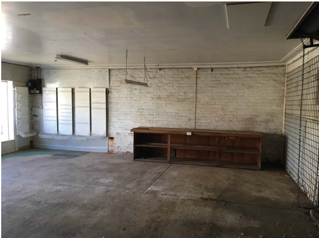
View of Brady's Saddlery, internal view (Image: Studio Two Architecture 26/06/2019)
