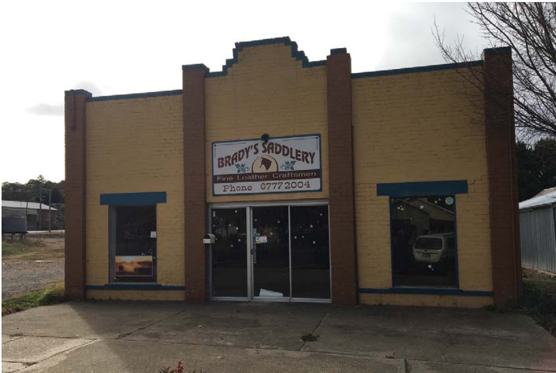
Shopfront entrance of Brady's Saddlery (Image: Studio Two Architecture 26/06/2019)
