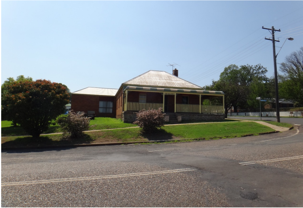
Image: Western elevation (Middle Street)
