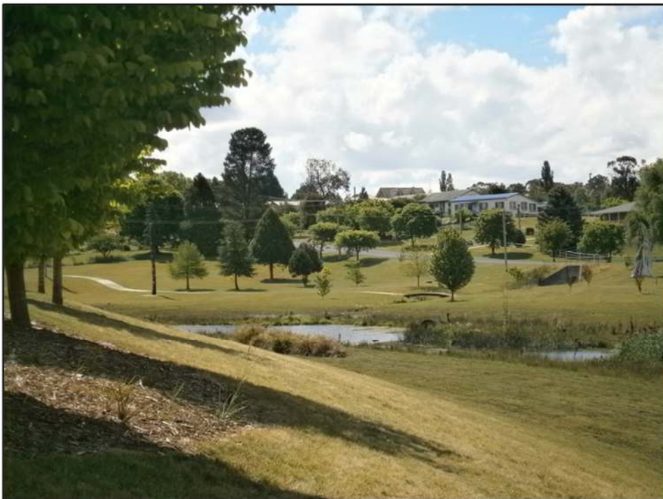
Apsley River Levee Banks
